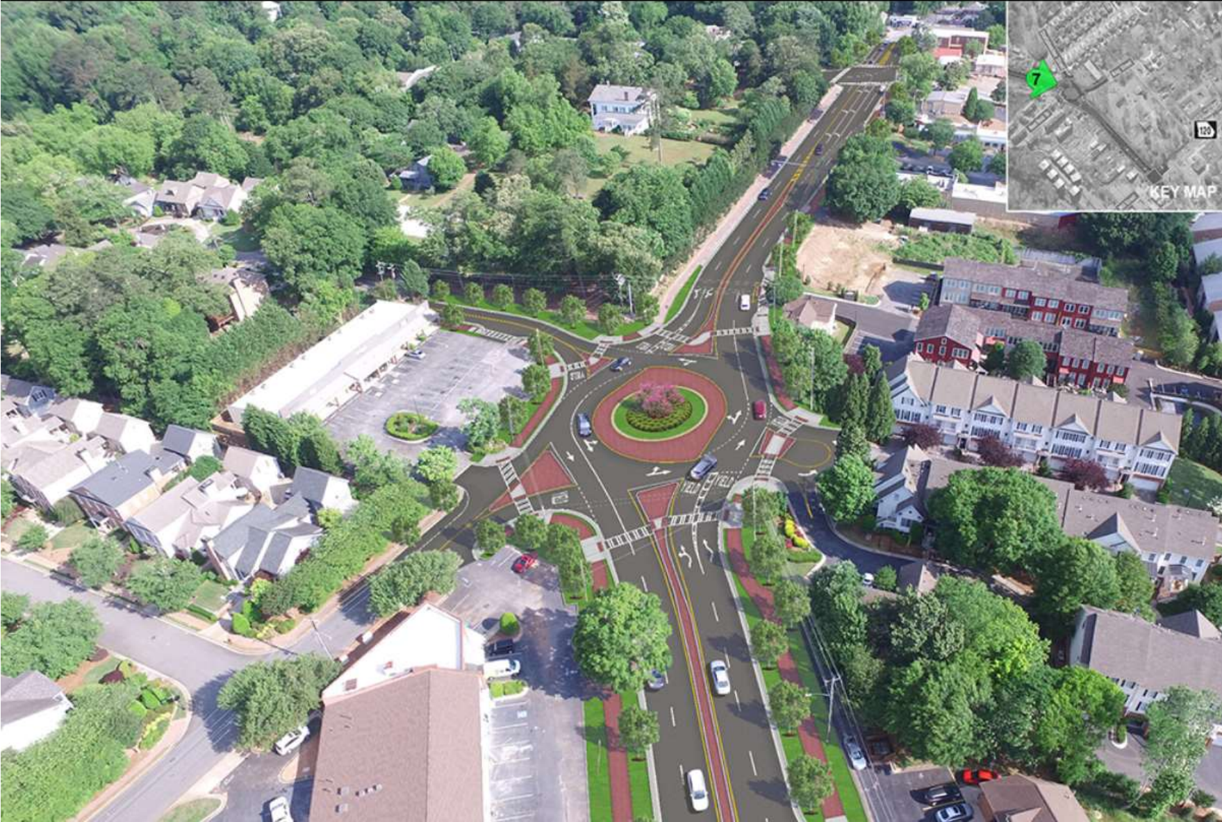
Location 7: NEW ROUNDABOUT ON SR-9 AT KING ST. (LOOKING NORTH)
