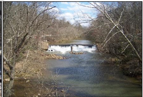
Big Creek Dam
