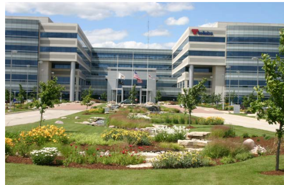
Figure 4-5 Office Complex – Naperville, IL
