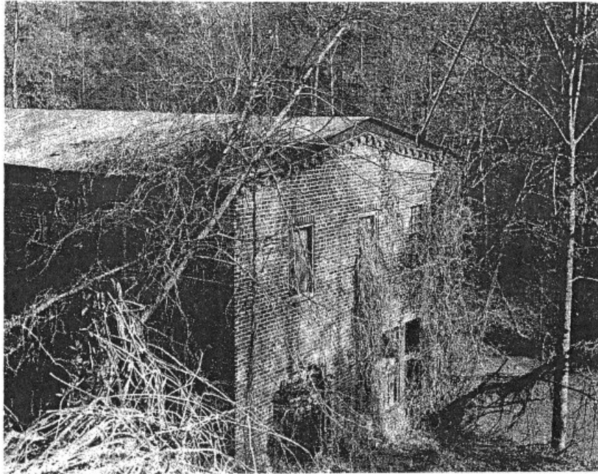
Plate 32 The Old Mill (note brick cornice design)
