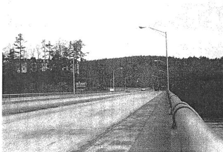
Plate 2 Chattahoochee River Crossing (looking north toward Roswell)
