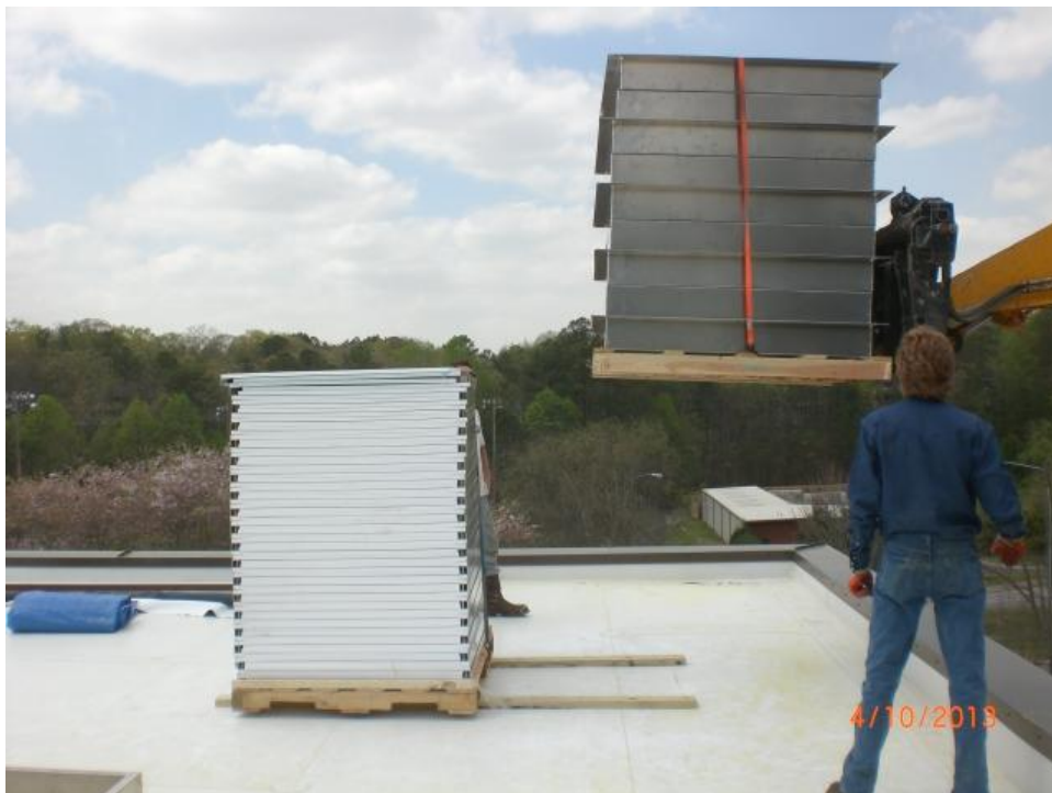
The skylight components and additional supplies were lifted to the roof.
