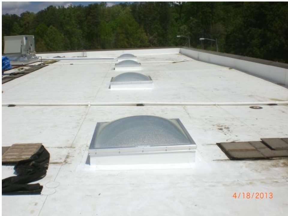
Finally, the skylight domes and frames were installed and mechanically fastened into position.
