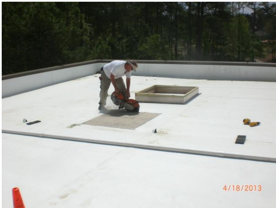
The location for each skylight was marked. The roof, insulation, and decking was then removed and disposed of off site.
