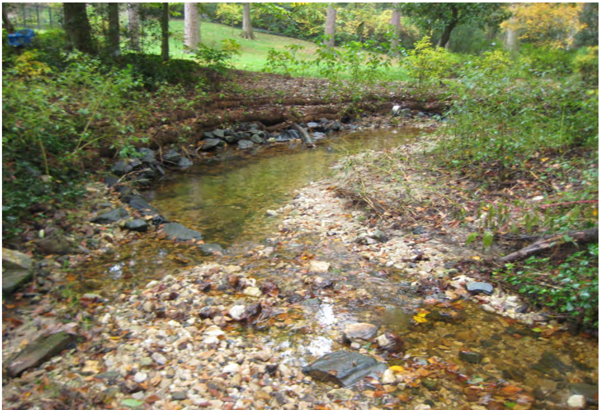
Coconut logs, live stakes, toe of slope protection and riparian restoration - Photograph courtesy of Register-Nelson Environmental Consultants.
