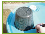
Trace a hole for the basket
