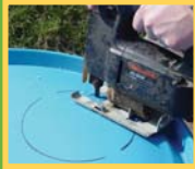
Cutting the top hole
