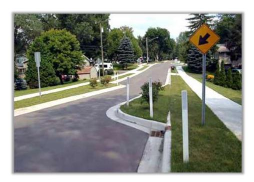
**Neck-Downs** – Physical modifications to the roadway that reduce or eliminate excessive pavement areas in order to encourage slower speeds. Neck-downs can be constructed from either the center of the roadway or from the outside (shoulder side) of the roadway or both. Neck-downs are often used in combination with chicanes or neighborhood entry features.
