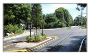
**Chicanes** – Physical modifications to the roadway that use a combination of horizontal curvature and lane narrowing to reduce speed, often creating a slalom effect. Chicanes can either maintain two-way traffic with narrowed lanes or reduce pavement width to allow for only one-way traffic time.
