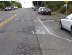
**Speed humps** are raised areas of a roadway that cause vertical upward deflection of travelling vehicles.
