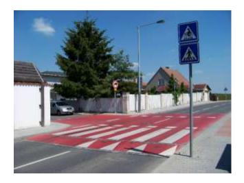
**Speed cushions** are raised areas, similar to speed humps, but do not cover the entire width of the roadway. They are designed to allow larger vehicles to "straddle" the cushions while smaller vehicles are vertically deflected. While some large vehicles and busses can pass with limited deflection, they can still affect emergency response times. They are more difficult to
