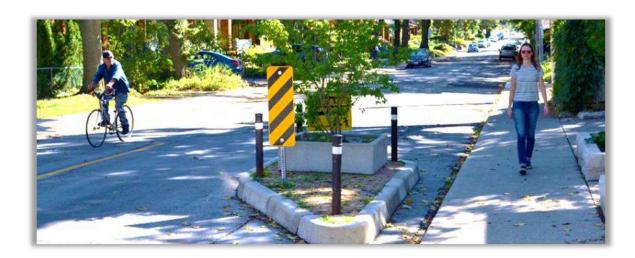
**Bulb-Outs (Curb Extensions)** – A special type of neck-down treatment that is primarily used to extend the sidewalks adjacent to a crosswalk further towards the center of the roadway, reducing the crossing distance and allowing pedestrians and vehicle drivers to see each other better when there is on-street parking or other sight obstructions.
